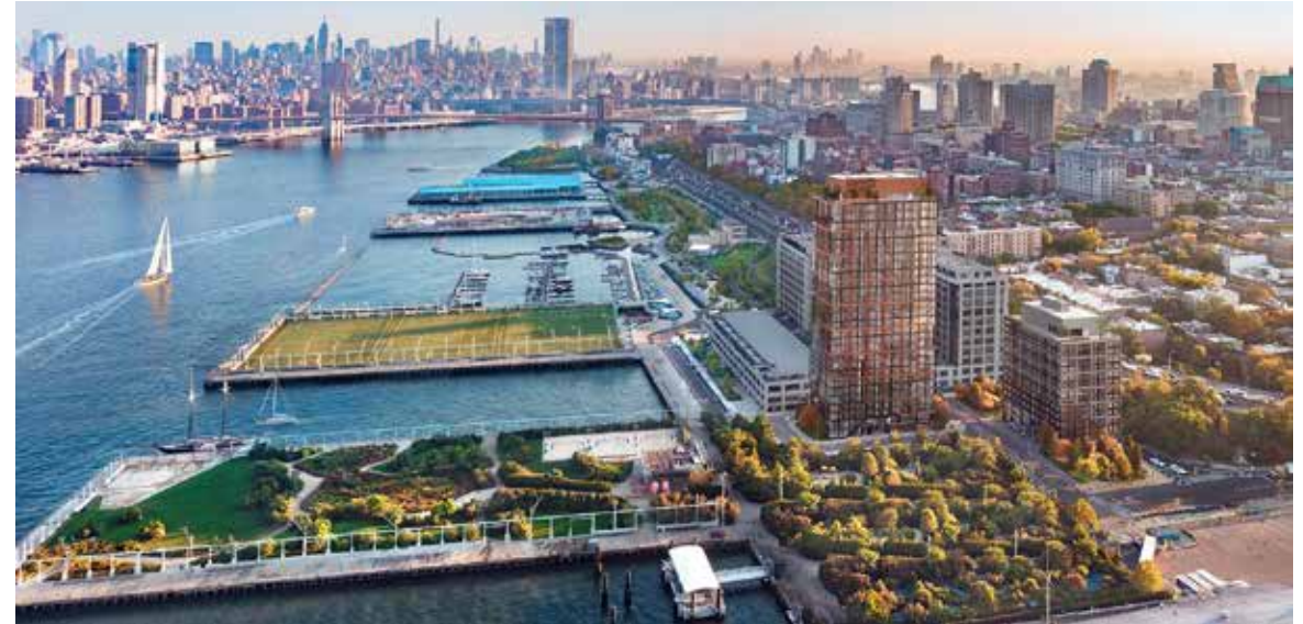
Brooklyn Bridge park, NY
