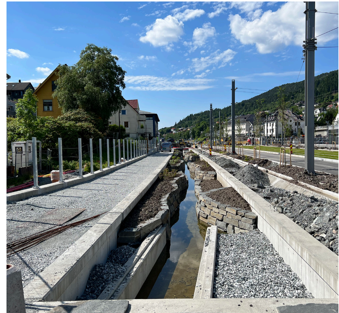
Foto: Kanalen as built. Sweco
