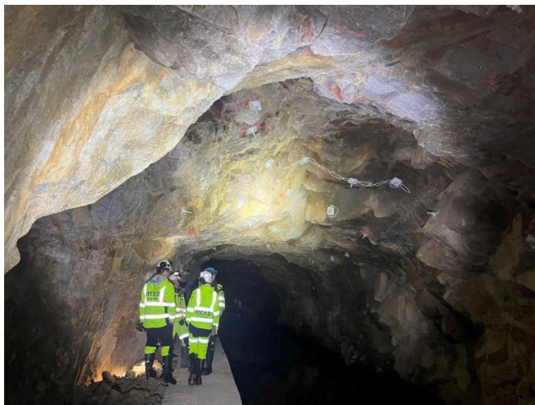
Figure 4-5: Chainage 30, picture taken towards south.
