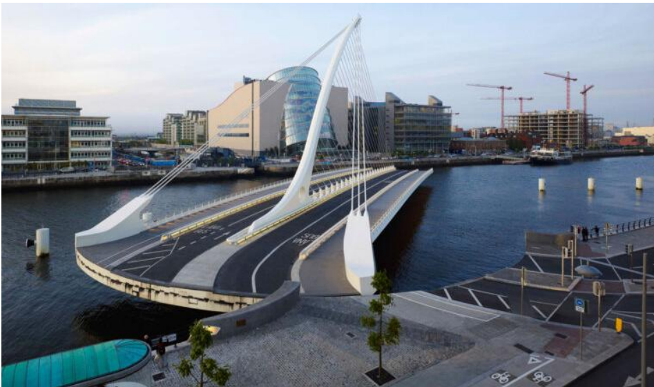
Figur 3-51: Svingebro. The Samuel Beckett Bridge (Dublin, Irland). Kilde: The Bridge Guy.
